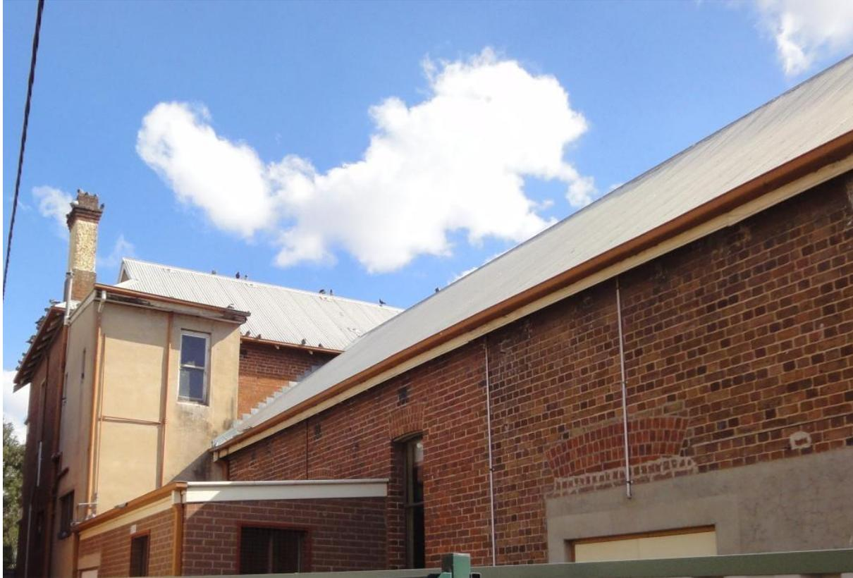
Additions over its life, including a side annex, are able to be identified at the rear of the building. Changes are visible in the brickwork where new work is cut in, including where a side door has been bricked up.
